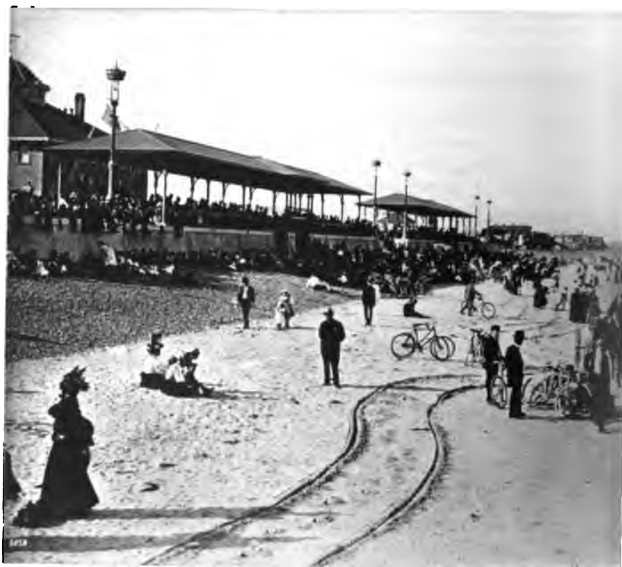
REVERE Terrace and shelters in front of the Bath-
